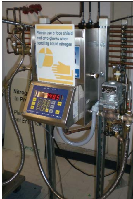
Low-Loss fill station controls. Middlesex installed this system at Genzyme to help curb excessive dewar handling.
