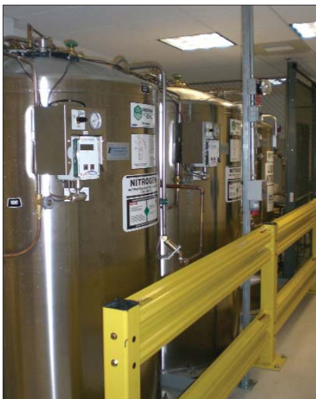
Two 1,500 liter nitrogen Perma-Cyls supply liquid nitrogen to Genzyme's Low-loss fill system. One 1,000-liter Perma-Cyl supplies nitrogen in gas phase throughout their building.
